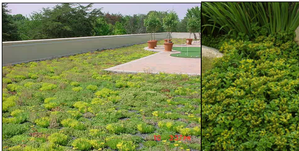
Figure 6.7: Sedum kamtschaticum applied to a green roof project ( greenroofplants.com ).
